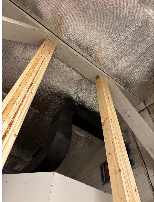
Pic: Two additional columns added.
