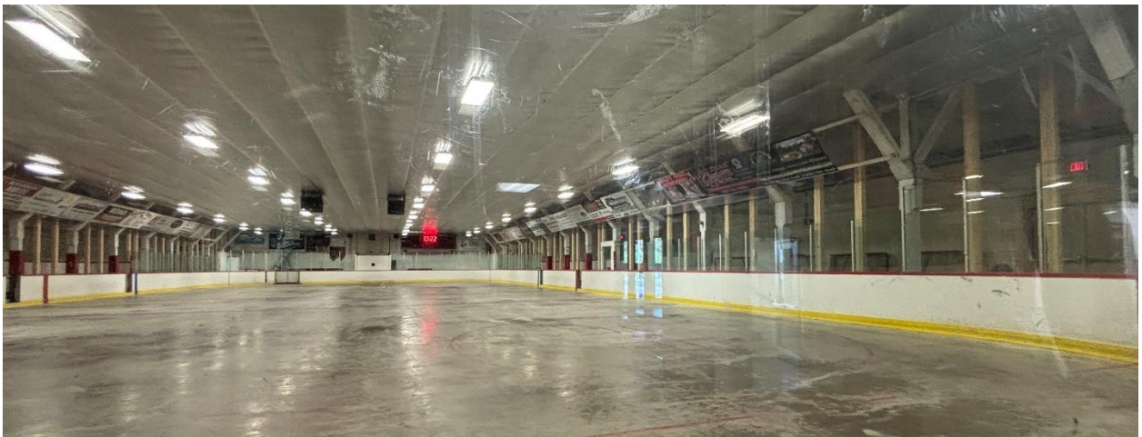
Pic: Interior of Arena – Extents of double columns.
