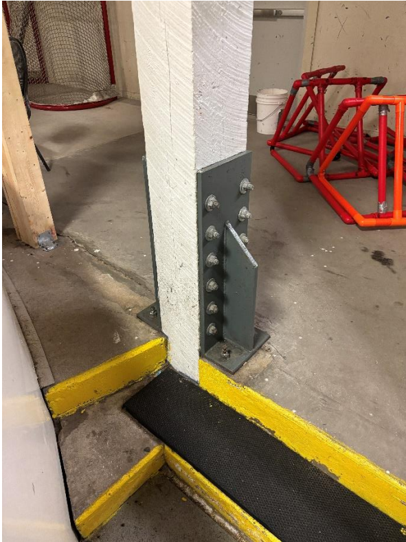
Pic: Steel reinforced post base.
